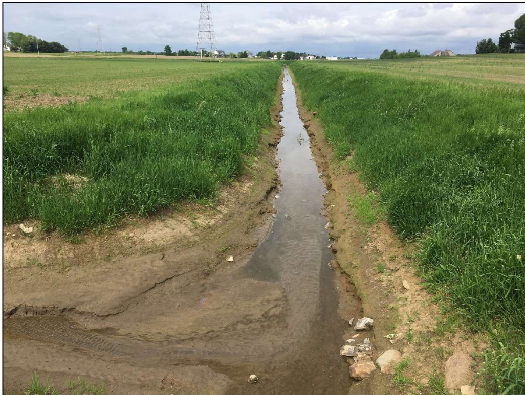
Stream FEL-1 (intermittent), facing downstream on May 29, 2020.
